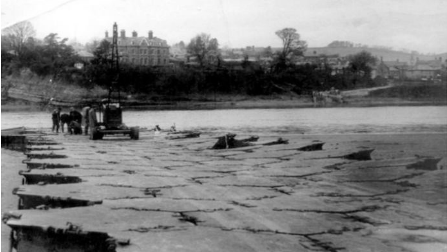
Harry Aldridge and Sons Building the bridge to Newnham
